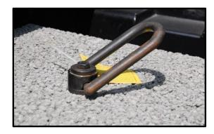
• Swivels shall be securely bolted snug to the slab. Check to ensure that the bolt extends the full depth of the lifting socket. To avoid damage to the surface do not over-tightened bolts. (An electric impact wrench with a 3/4" socket is the most efficient way to attach and remove the swivels).
