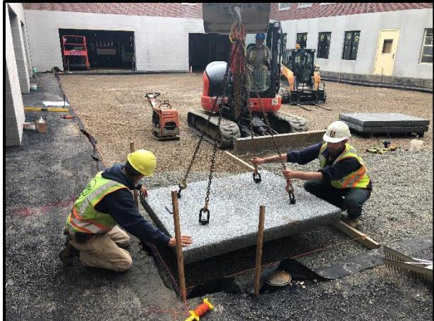
Stormcrete® is a modular precast porous concrete system which provides a reduced-risk alternative to poured in place porous pavements. Routine operation and maintenance (O&M) procedures are similar to that of conventional pervious pavements. However the use of Stormcrete® provides the security of knowing that the slabs may be easily lifted for maintenance and subsurface repairs. Individual or multiple Stormcrete® slabs may also be removed and replaced or reused.
