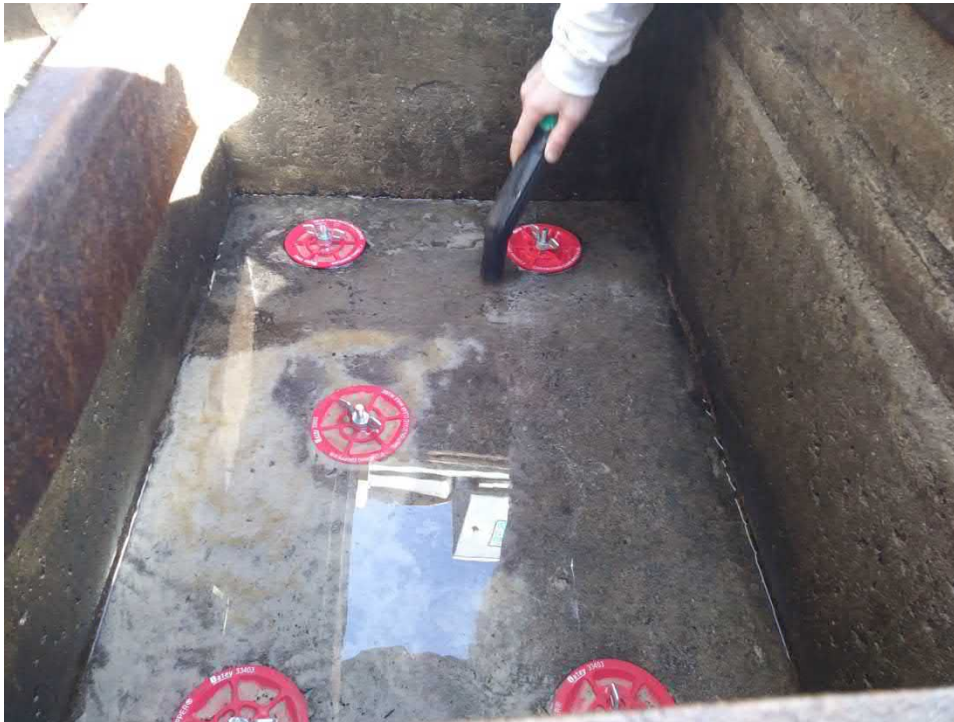
Figure 46. A wet-dry vac was used to remove sediment from the bottom of the Bloomington sump. The red plugs were inserted to seal infiltration holes in the slab to limit sediment loss.
