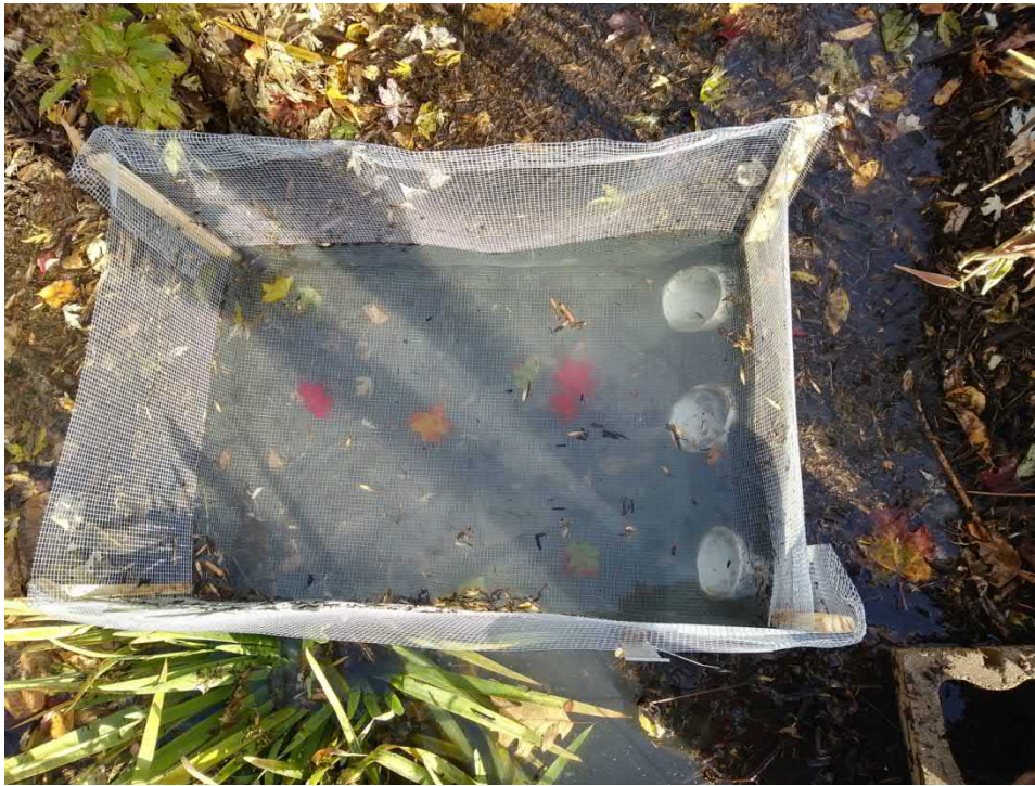
Figure 23. Gross solids containment area at Bloomington field site. Flow from the shallow sump box enters the bioretention basin through the three pipes at right.
