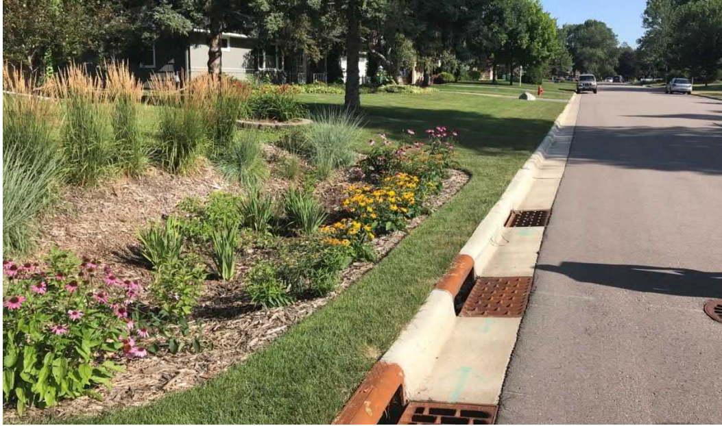
Figure 5. Queen Avenue rain garden in Bloomington, looking north. The inlet to the pretreatment device is through the furthest curb grate. The gutter low point is between the middle and bottom catch basins.
