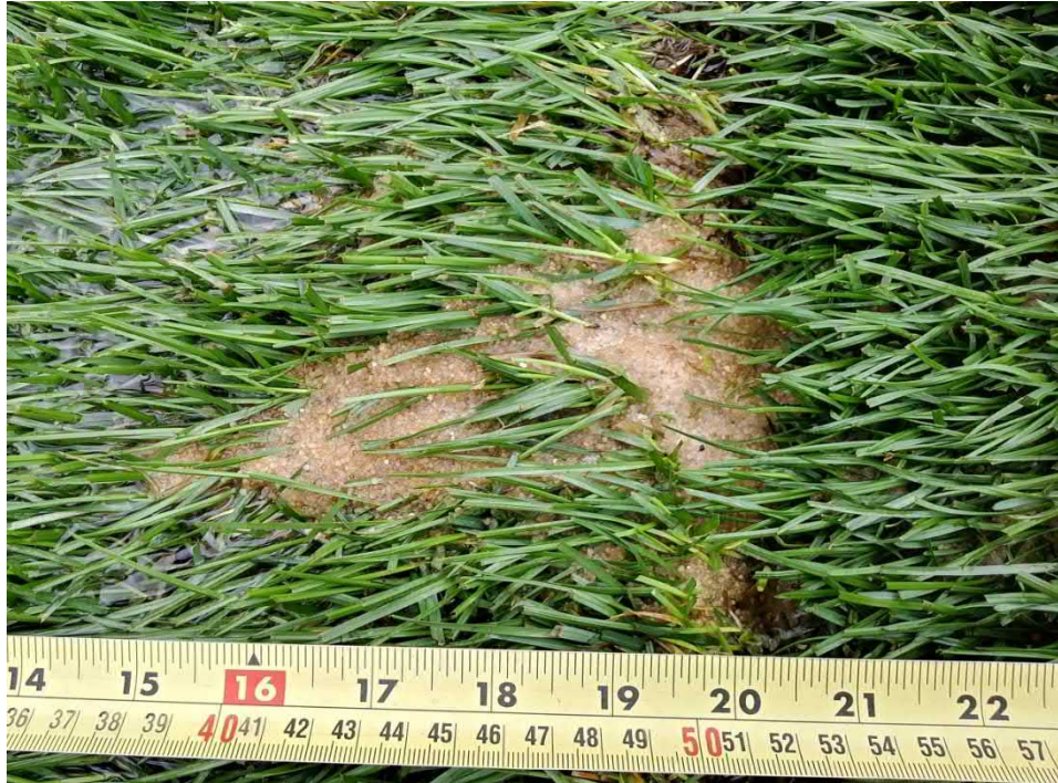
Figure 52. Sediment accumulation near the horizontal seam between sod sections in the GLI. Flow was right to left.
