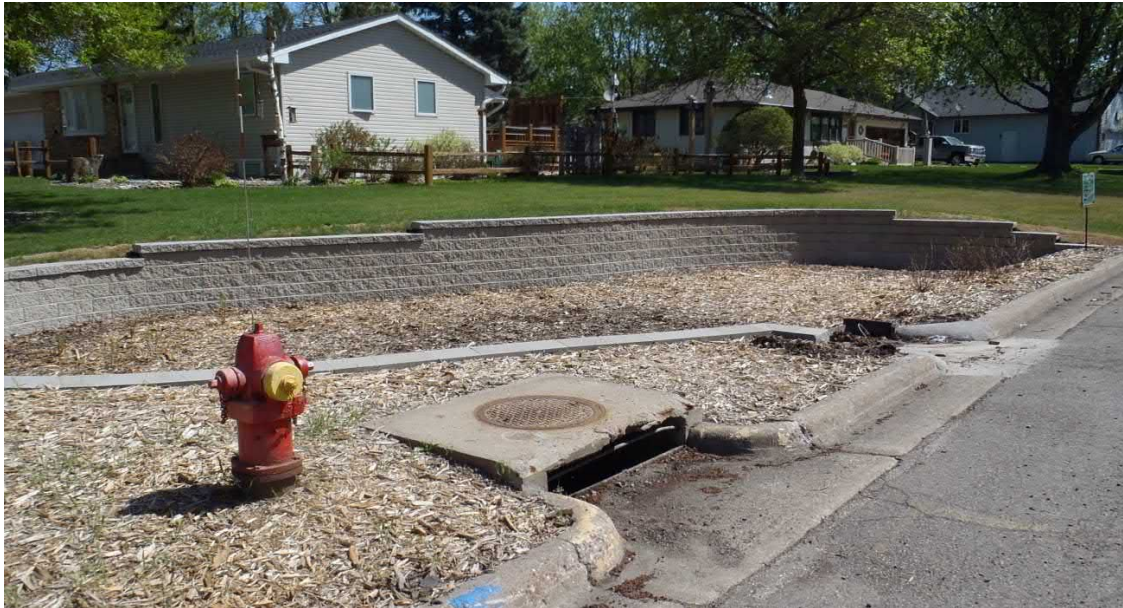
Figure 1. Photo of the Anoka site in May 2018, prior to testing. Gutter flow along 38 th Lane is from right to left in the photo, encountering the basin inlet before the large catch basin nearest the fire hydrant.
